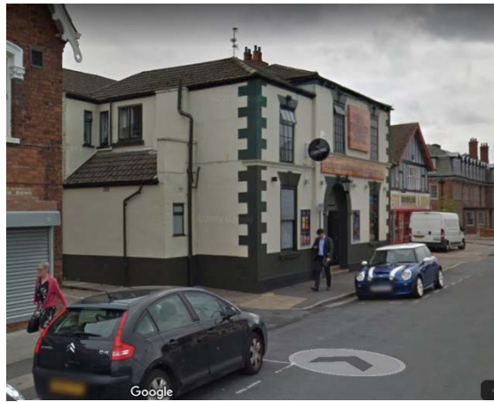
Current day view of County Hotel, Brighowgate. Note the change in roof level and remains of chimney breast
