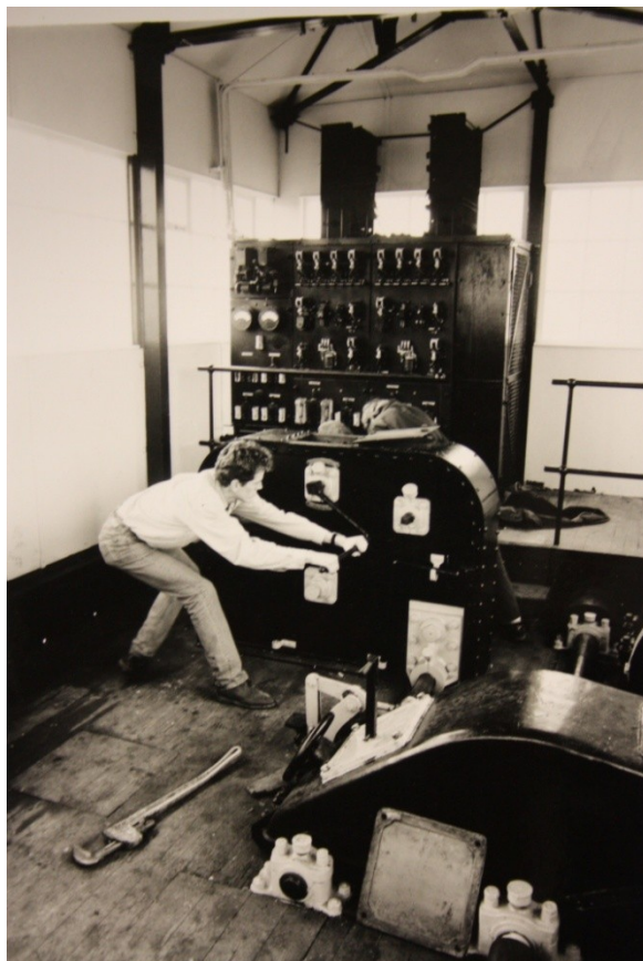
Plate 4: Photograph of the bridge being raised by means of hand winch
