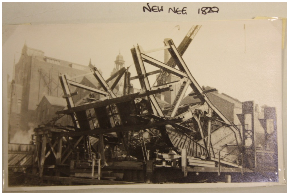
Plate 3: Photograph of the new Corporation Bridge under construction in 1925
