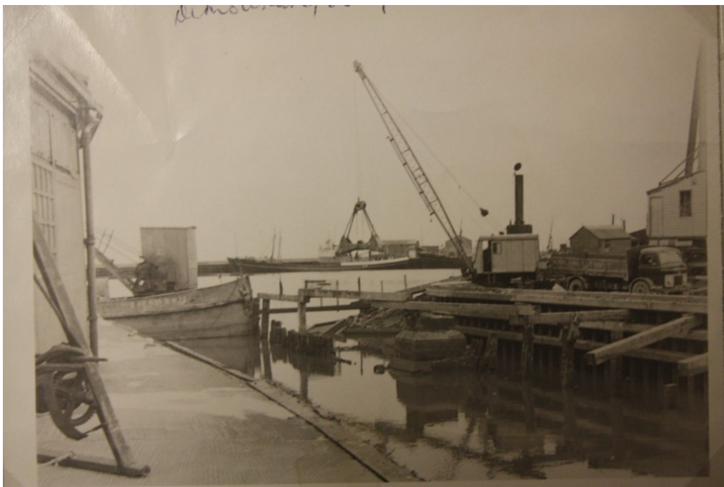
Plate 2: The Old Corporation Swing Bridge photographed in the course of demolition circa 1925
