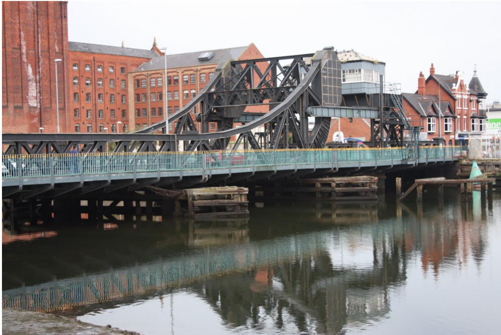
Plate 7: View of bridge showing steel and cast iron structure, bridge house and cantilever footways
