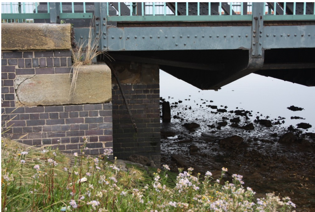
Plate 8: View of blue brick and ashlar stone abutment
