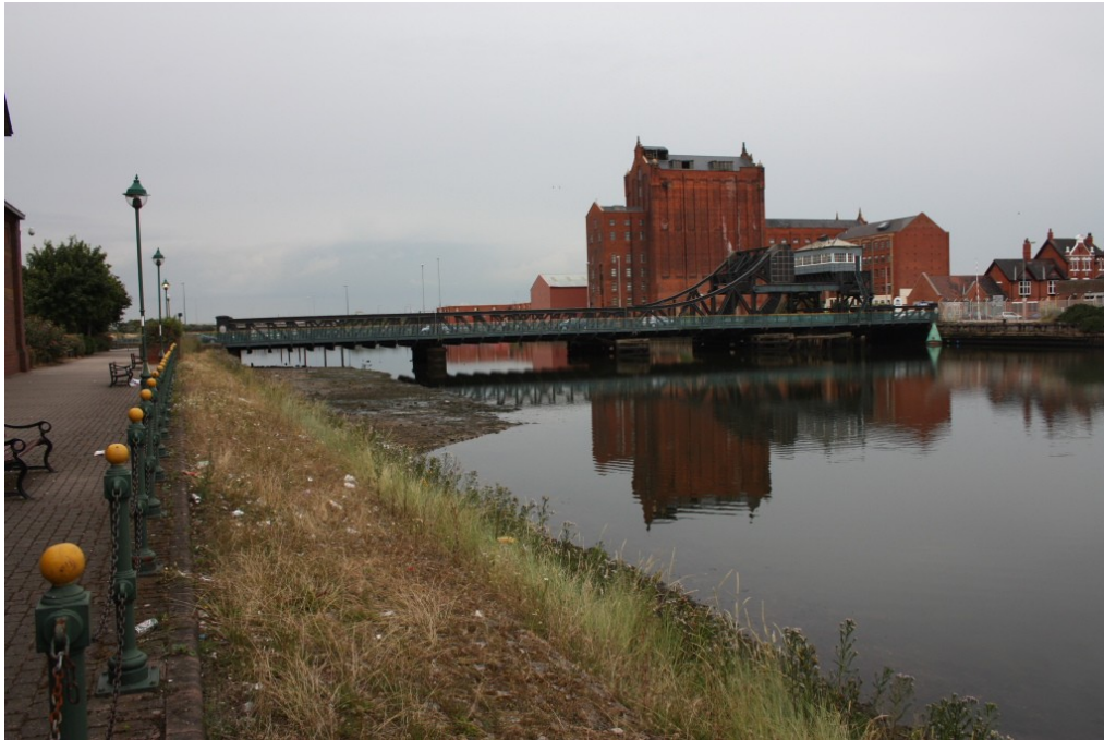
Plate 1: General view of Corporation Bridge looking along Alexandra Dock from the south. Note the former Victoria Flour Mills beyond.
