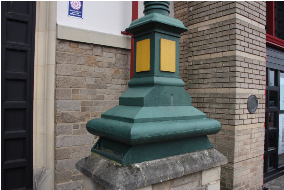
Plate 14: Detail of the base of one of the original cast iron lamp columns, re-erected at the National Fishing Heritage Centre in 1991
