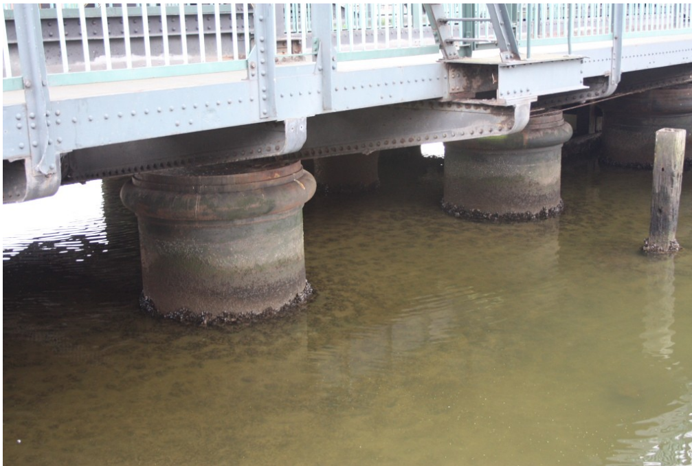
Plate 9: View of cylindrical piers supporting the bridge
