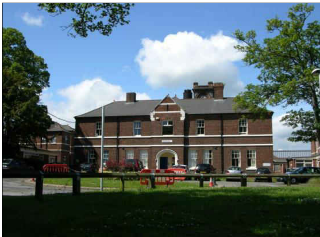
Central Administrative Block
