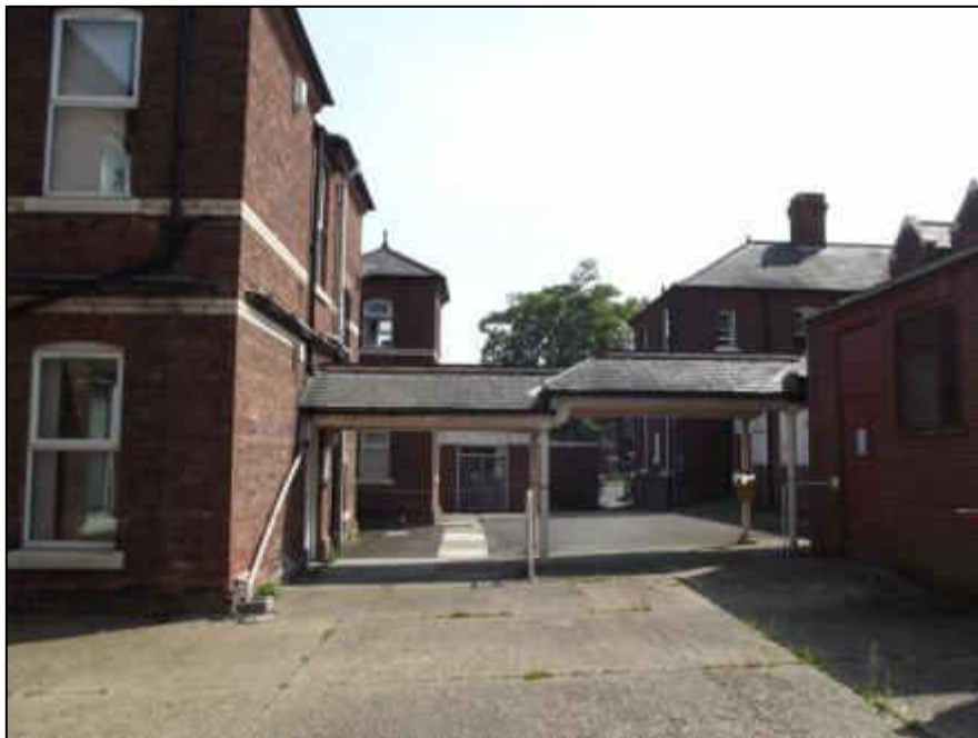
One of the covered walkways between buildings
