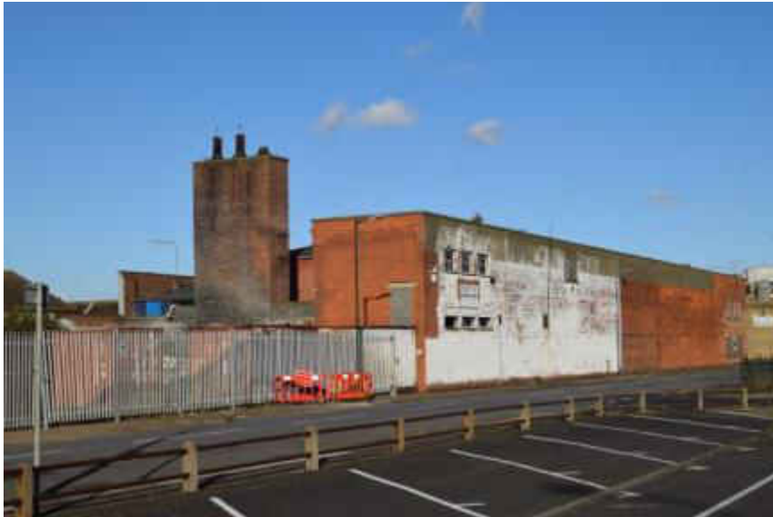
Compass House from the south west, showing the smoking tower
