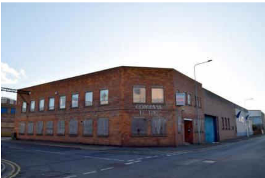
Compass House from the north east
